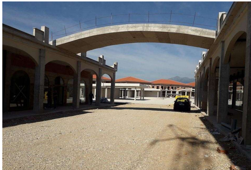
Figure 7: The first phase of the construction of bridges within the complex
