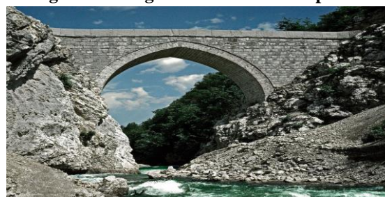
Figure 1. Bridge from the Ottoman period
