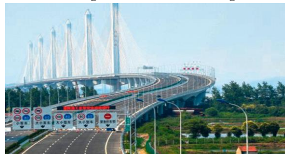
Fig. 2. A modern bridge built on the basis of knowledge and modern technologies
