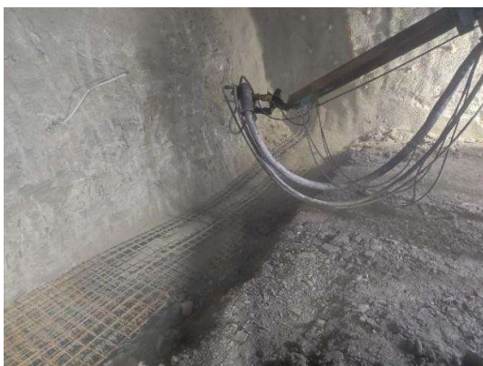
Figure 6. Installation of shotcrete on pre-reinforced II reinforcement zone/temporary invert (photo. N. Halilbegović, 2024)
