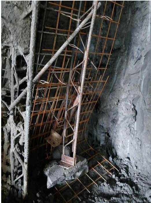
Figure 8. Detail of the "elephant's foot" installation (photo: N. Halilbegović, 2024)
