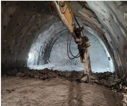
Figure 5. Excavation of the temporary invert (photo. N. Halilbegović, 2024)
